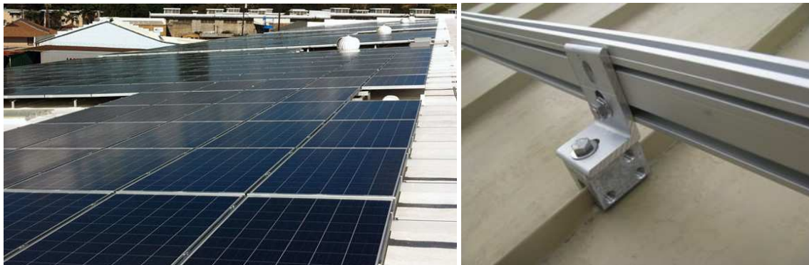
Fig. 2: A mounting clamp system shown for installation of solar panels on the roof structure. Various methods of mounting are available, including struts and interference clamps which cause no holes or punctures to a rooftop. Easements and clearance for other gear installed on a roof are made by removing panels from the module array. An example of an interference fit clamp is shown in the right.
